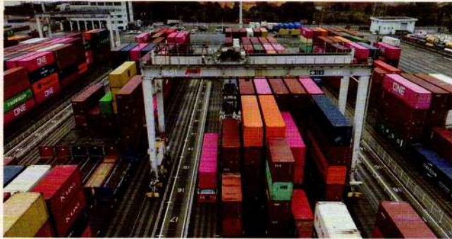
自動化RTG(Rubber Tired Gantry crane)
